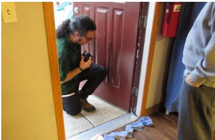
Left Photo: Energy Program Coordinator Marcus Ricci assesses a failed door threshold.
