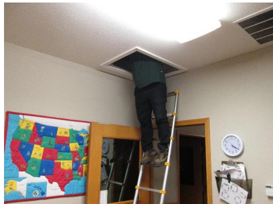
Checking attic insulation levels.
