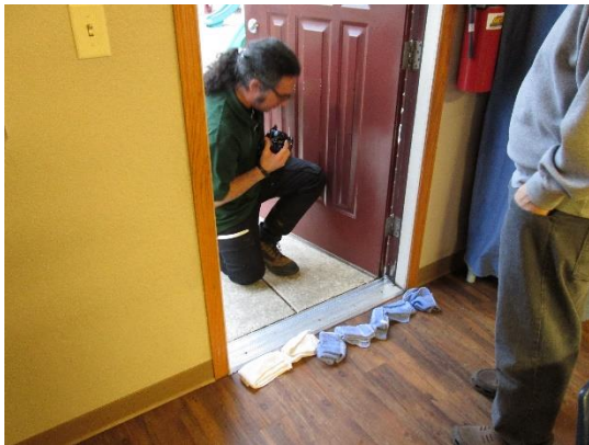
Checking door seal and threshold.
