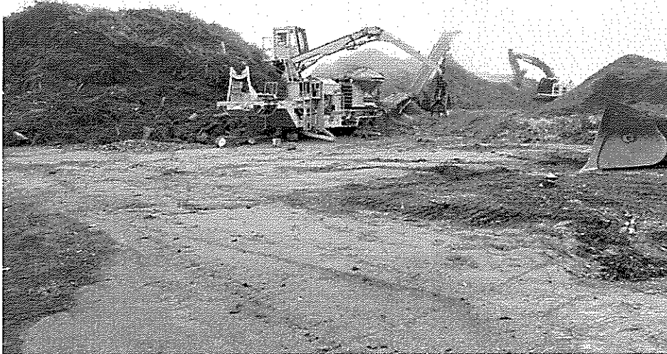
Processing brush into mulch
