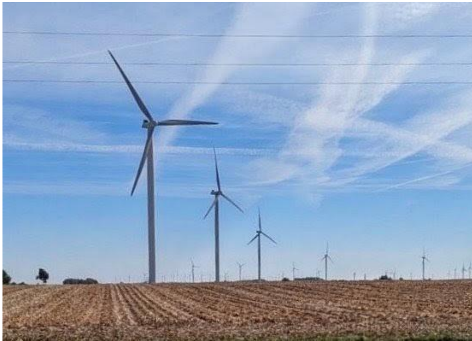
Figure 1.6: Twin Groves Wind Farm, one of many examples of McLean County's leadership in renewable and clean energy. (Photo supplied by EAC, 2023)
